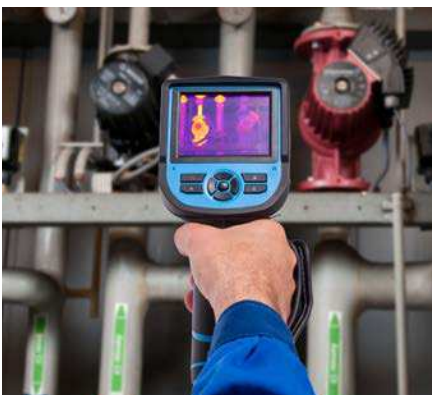
3 Perform thermal imaging with SKF Thermal Camera TKTI series
