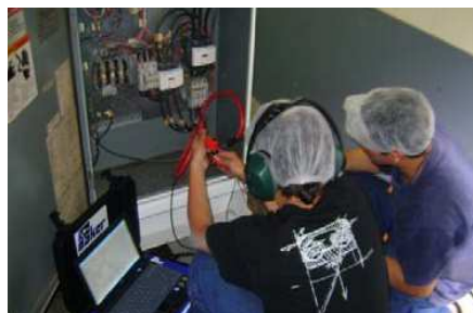
Checking electric motor performance with the SKF Dynamic Motor Analyzer.
