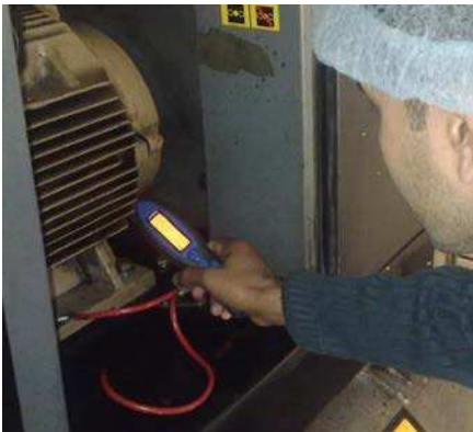
1 Monitor vibration with SKF Machine Condition Advisor, CMAS 100-SL
